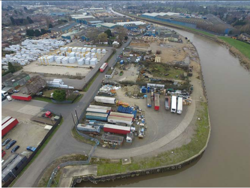
Above - General view of Wisbech Port – looking south
